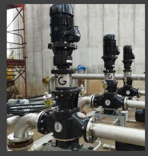
Grinders upstream of progressive cavity pumps to prevent damage and clogging from solid bodies.
